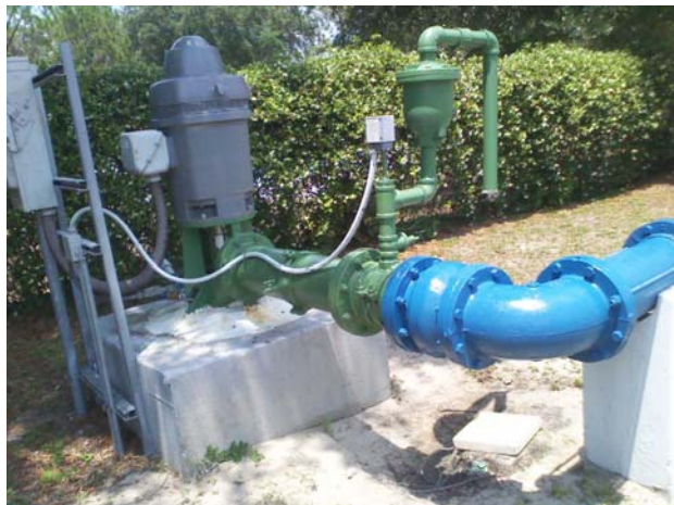
Jacob WTP after painting and rehab.
