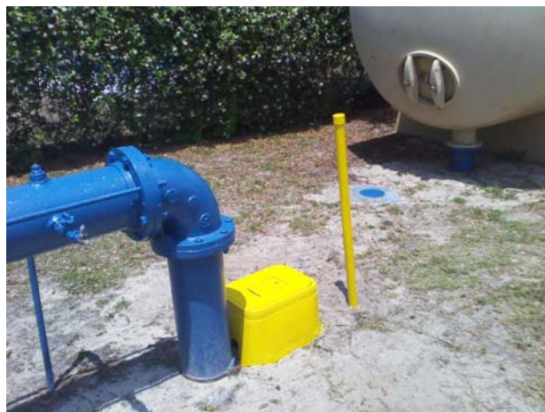
Jacob Water facility chlorine injection rehab completed.
