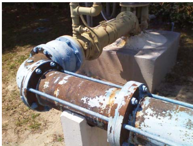
Jacob WTP before painting and rehab.
