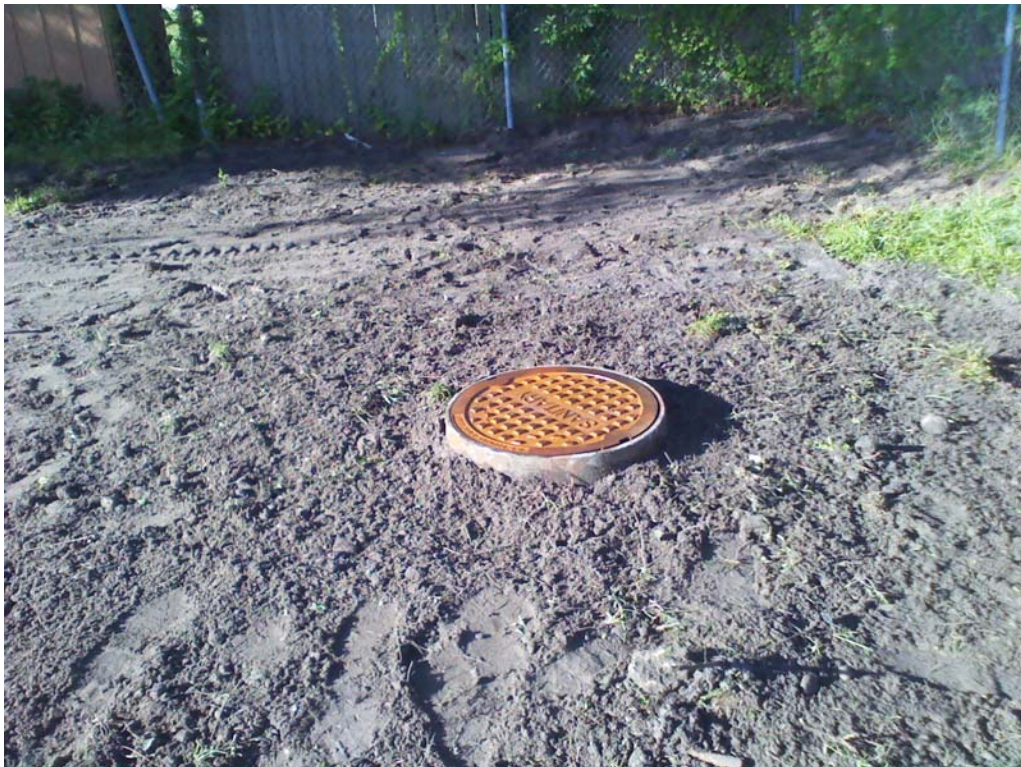
Site after manhole repair completed.
