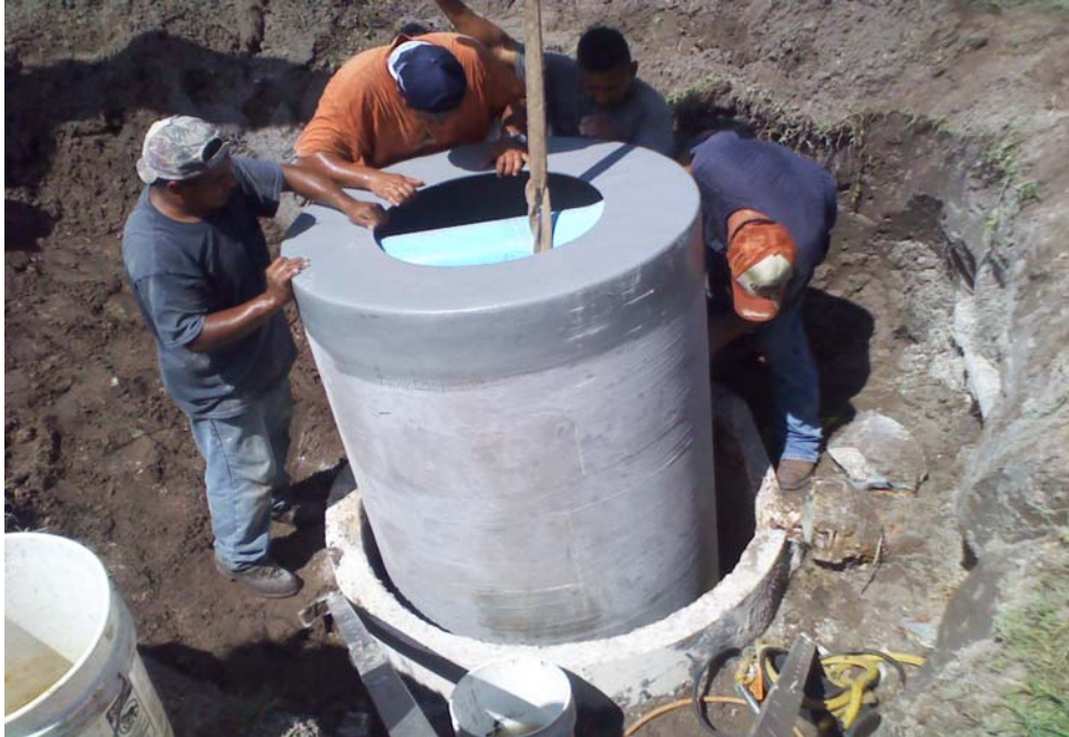
Liner being installed into failed manhole.
