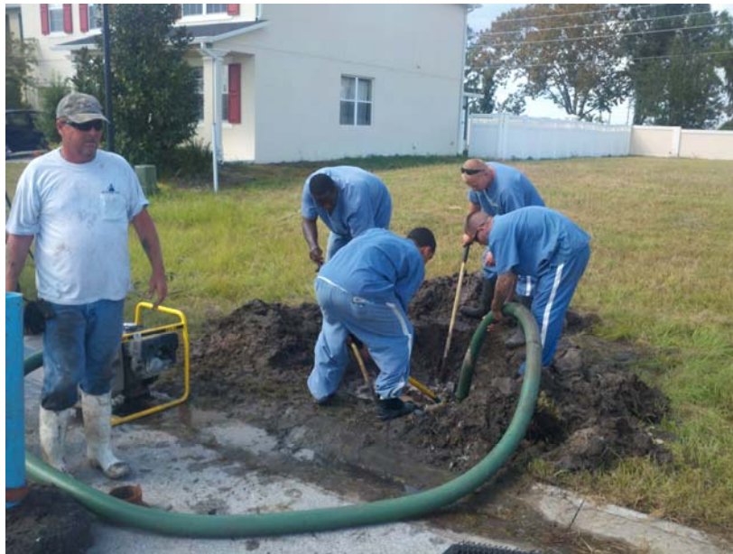
Water line repair at Hinsdale Heights in Fountain Park.
