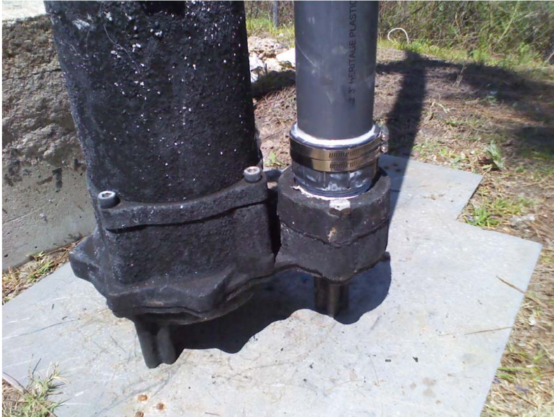
New riser pipe installation at Golden Gate Liftstation.
