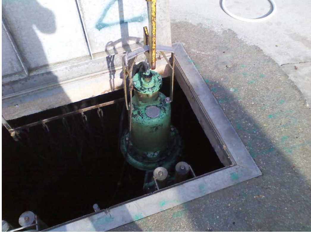
Dropping liftstation pump back into station after servicing.
