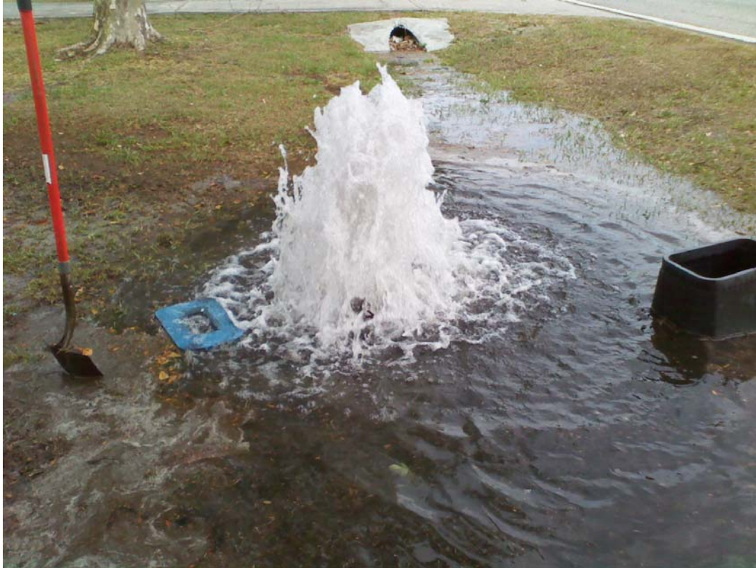
Water Leak over the weekend.
