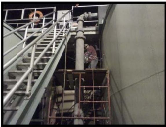
Influent tie-in for the new headworks.
