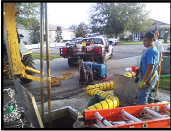
Working on liftstation rehabilitation.
