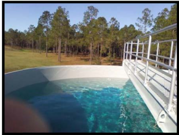
Leak testing of new EQ tank at Cardinal Hill.
