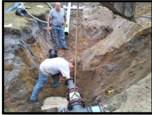
New force main connection at Voyles Loop.
