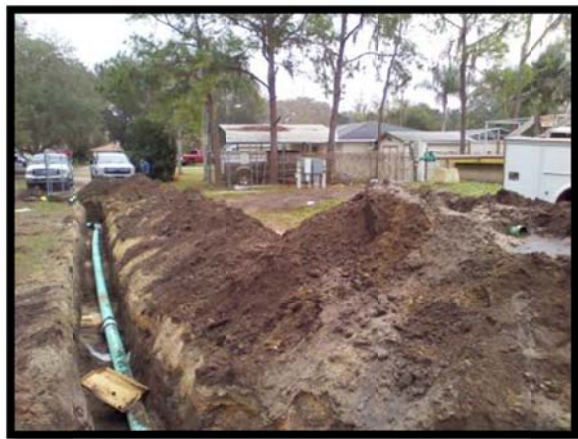
Final sewer main tie-in at Mt. Olive WWTF.
