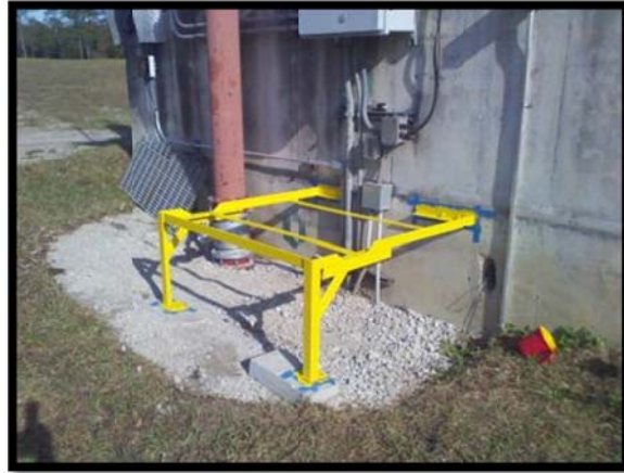
Installed new access platform at Cardinal Hill WWTF.
