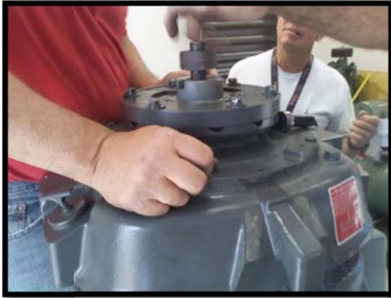
Working on Matt Williams WTP.
