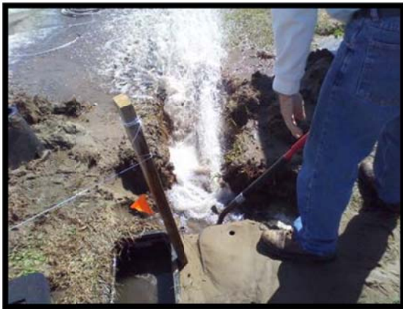
Service line leak repair on Motor Coach Dr.
