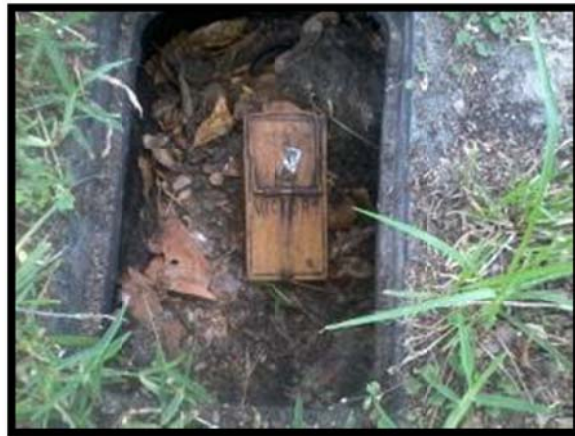
Present left in meter box by friendly customer.
