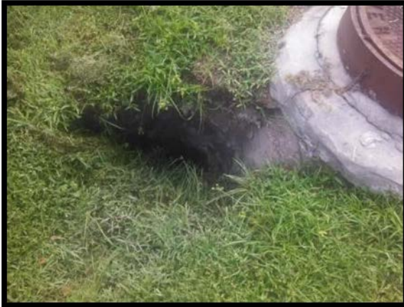
Sinkhole at manhole on Sarah and Samaritan, and plumbing company using camera to identify issue.
