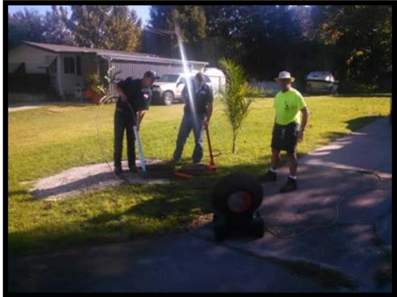
Sinkhole at manhole on Sarah and Samaritan, and plumbing company using camera to identify issue.
