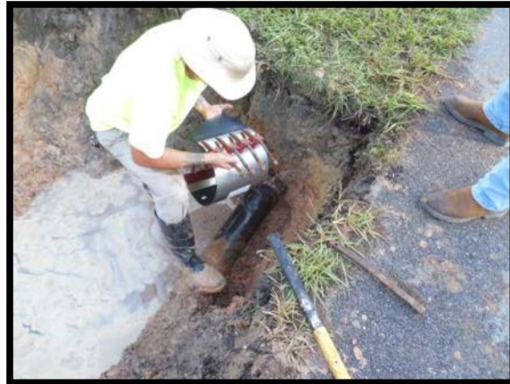
Cracked 6 inch water main on Oak Ave.
