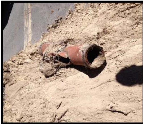
Broken sewer line and water line.
