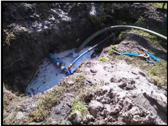
Water leak repair at the end of water line.
