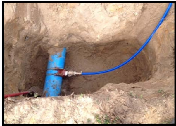
Water main tap for service relocation on Meandering Way.
