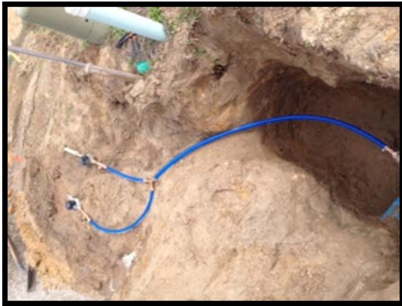
Water main tap for service relocation on Meandering Way.
