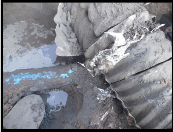
Water line break on Golden Gate Blvd.
