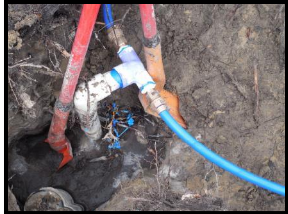
Water line repair.
