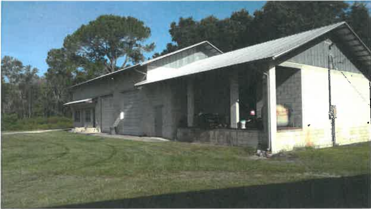
Office/Service Garage Building
