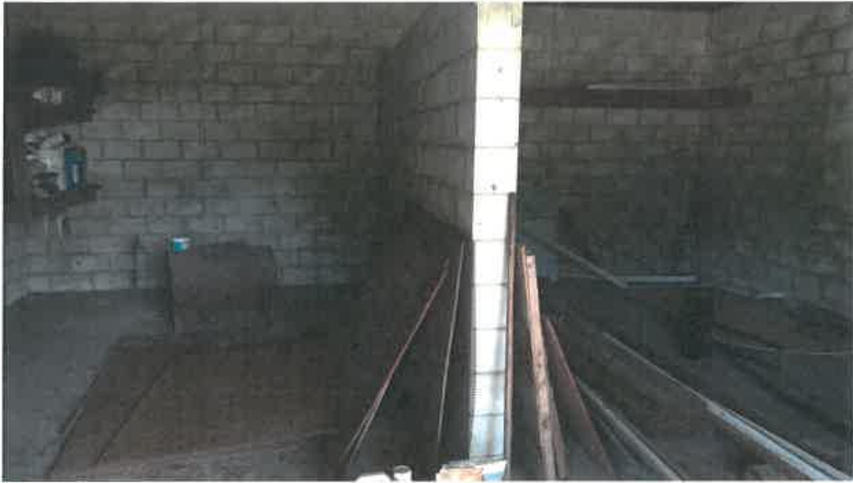
Interior of Service Garage
