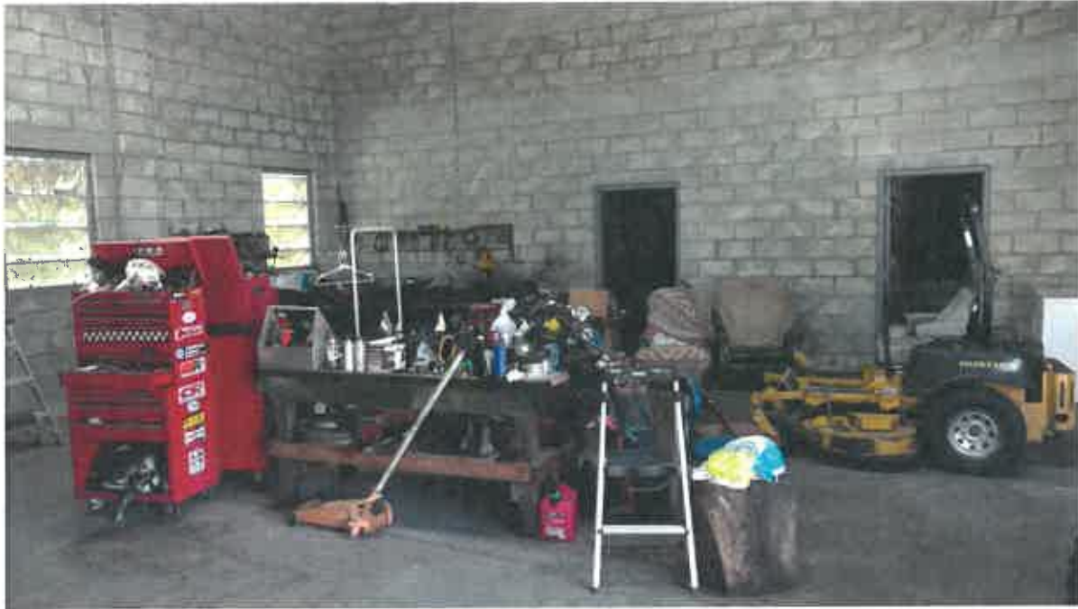
Interior of Service Garage
