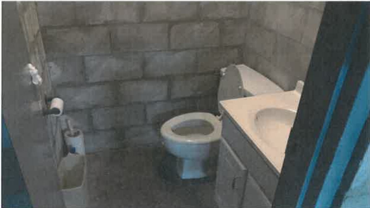
Interior of Office/Service Garage
