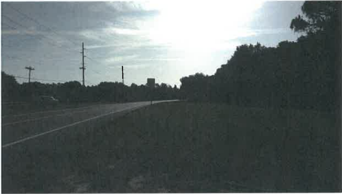
State Road 33 N – Looking East
