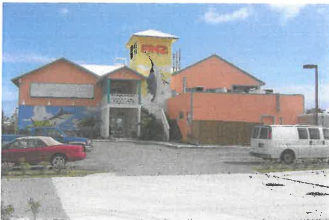
Martin County Finz Restaurant Infrastructure CDBG Economic Development
