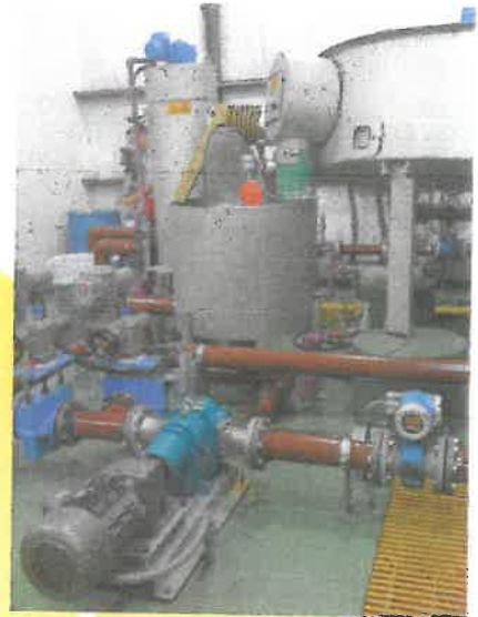
City of Starke WW Tertiary Treatment CDBG Neighborhood Revitalization/Clean Water SRF
