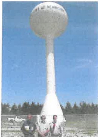
City of Newberry Elevated Water Tank CDBG Economic Development
