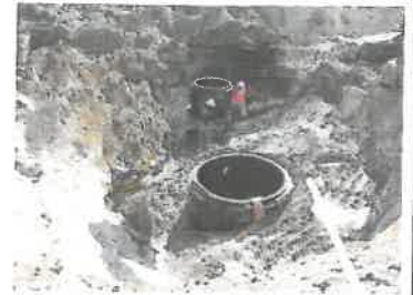
City of Monticello Sewer CDBG Grant
