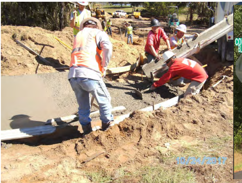
FDOT SCOP NORTH FRANCIS STREET & MACGILL STREET PAVING
