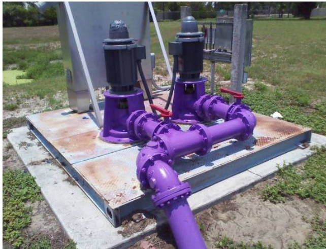
Hwy 33 Spray Field pumping station rehabilitation
