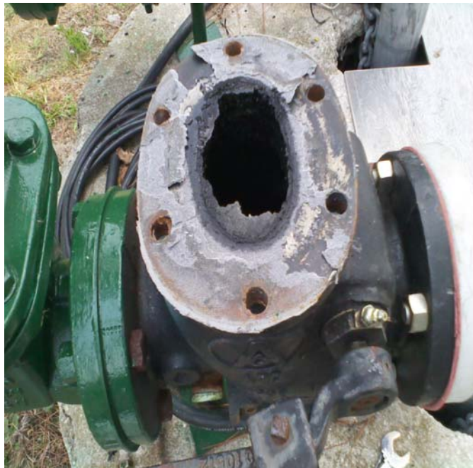
Check valve cleaning and maintenance at Golden Gate lift station
