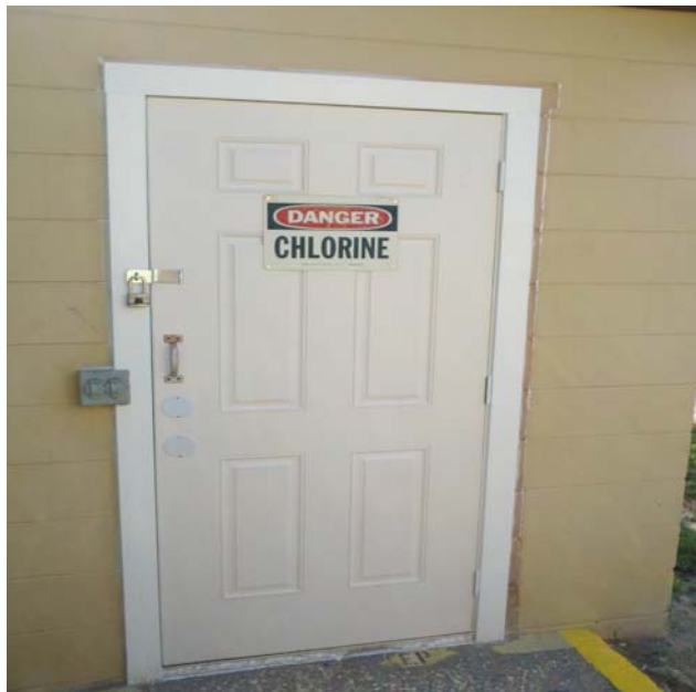
New door installed for chlorine room at Jacob WTP
