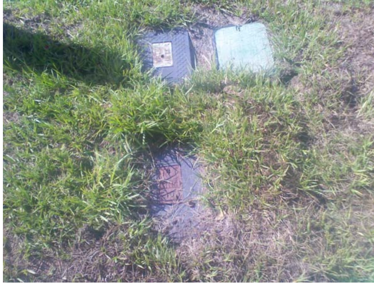
New meter installations.
