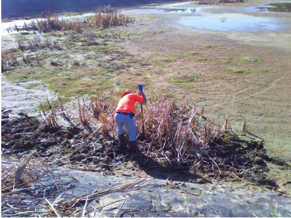
Removing vegetation from Cardinal Hill WWTP reject pond.
