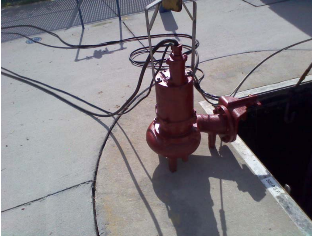
Repaired pump at Two Ponds Rd.
