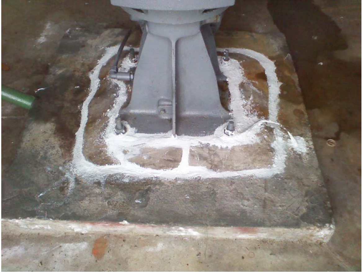
Well seal repair at the Commonwealth WTP.
