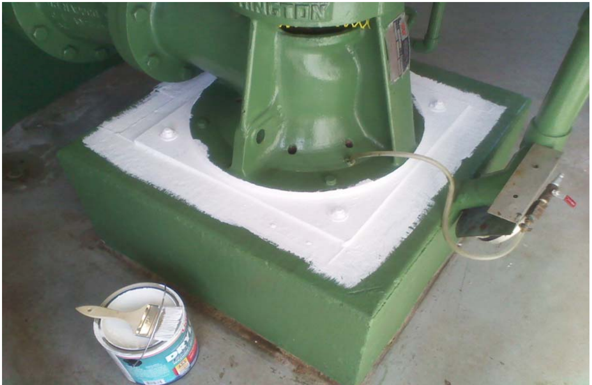
Special paint designed to re-enforce the well seal.
