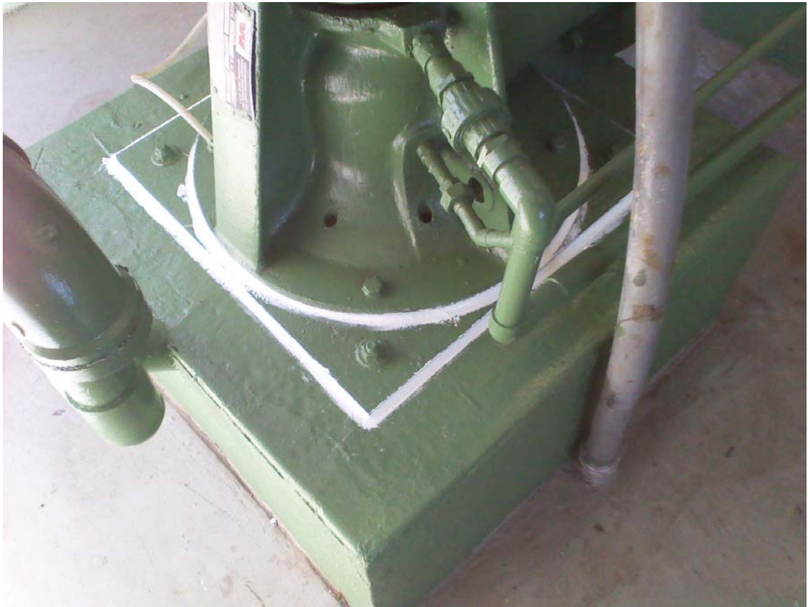
Well seal repair at the Matt Williams WTP.
