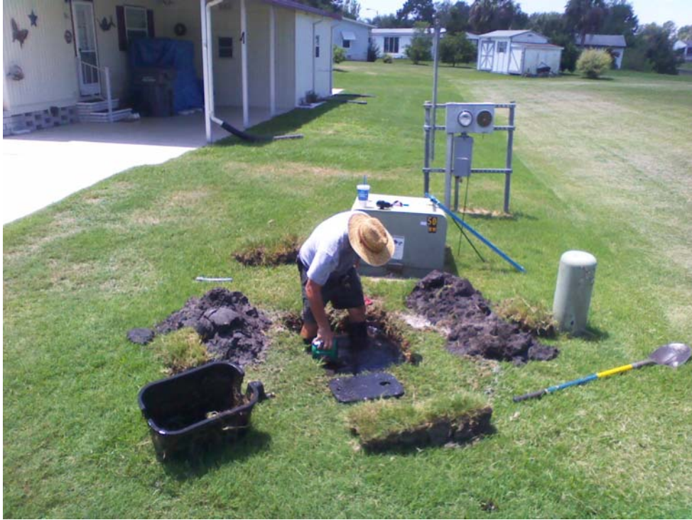
Water leak being repaired.
