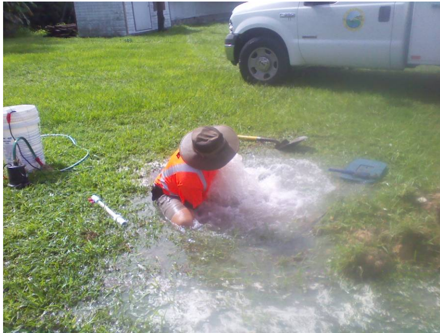
Howard working on water leak just off Berkley Rd.
