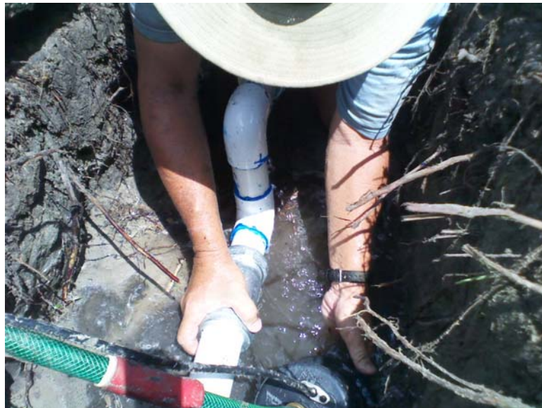
Water line repair coupling being installed.
