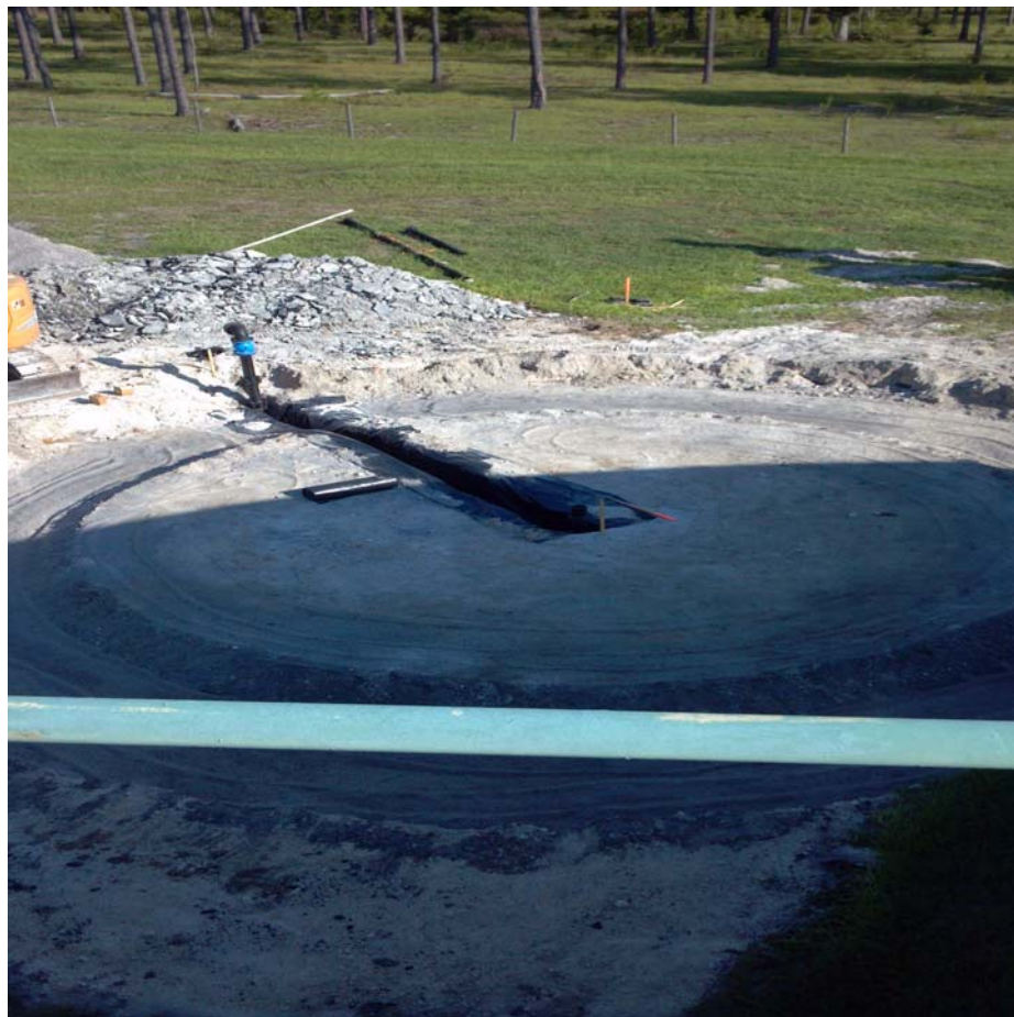
Foundation site for new treatment tank.
