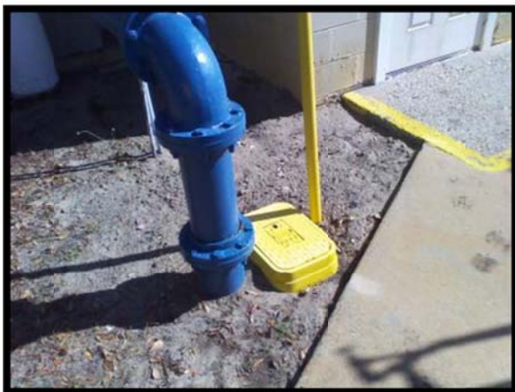
Repaired cl2 injection point at Mt Olive WTP
