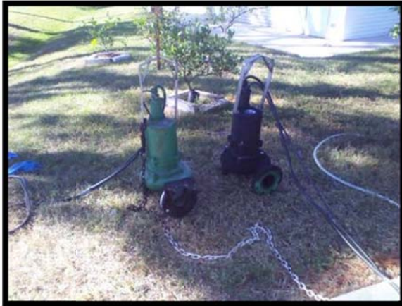
Pumps swapped at Liftstation #10.
