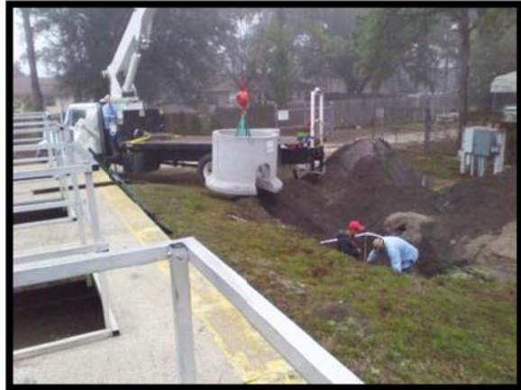
Vault being installed over new flow meter.
