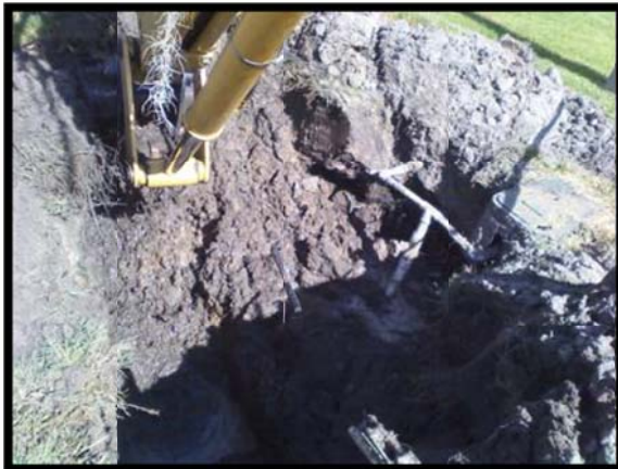
Water line repair on N. Island View Circle.
