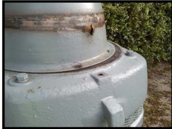
Top brake and ratchet gear came apart on 75hp motor at the Jacob WTP.
