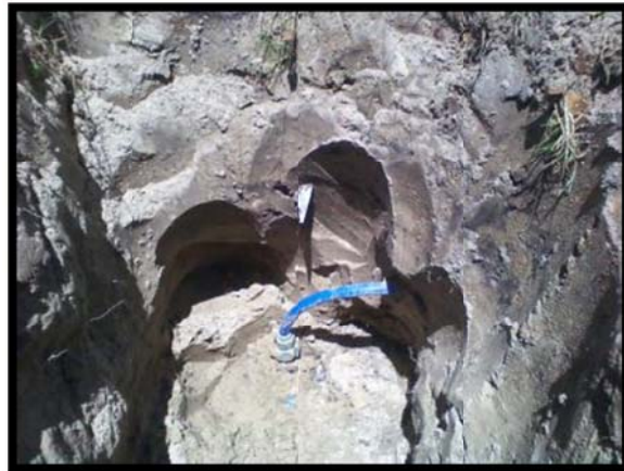
Typical new service connection tap.
