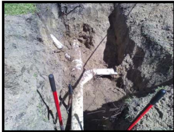
Sewer line repair on Golden Gate Blvd.
