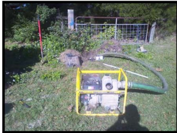
Service line leak repair.
