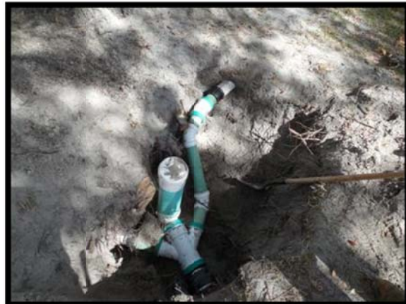
Sewer lateral repair on Jericho Ave.
