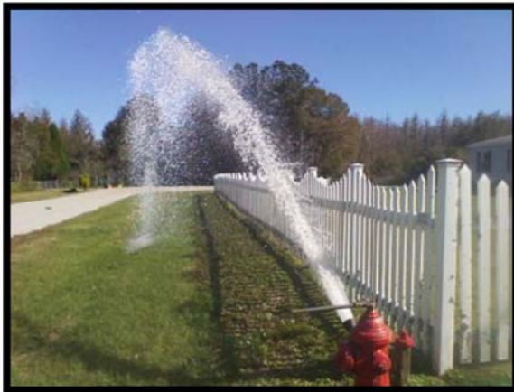
Hydrant Flushing.
