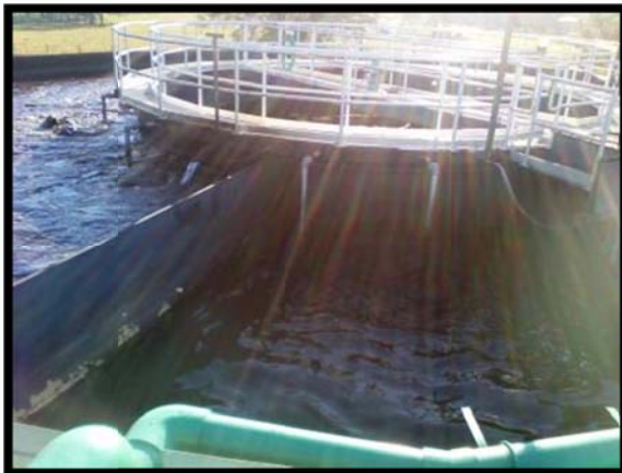
Early morning at Cardinal Hill WWTF.
