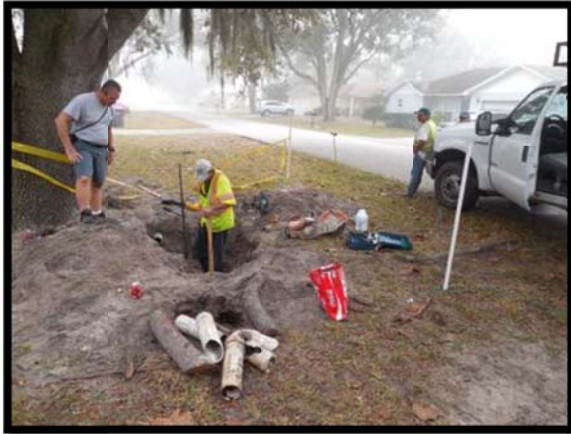
Sewer lateral repair on Jericho Ave.
