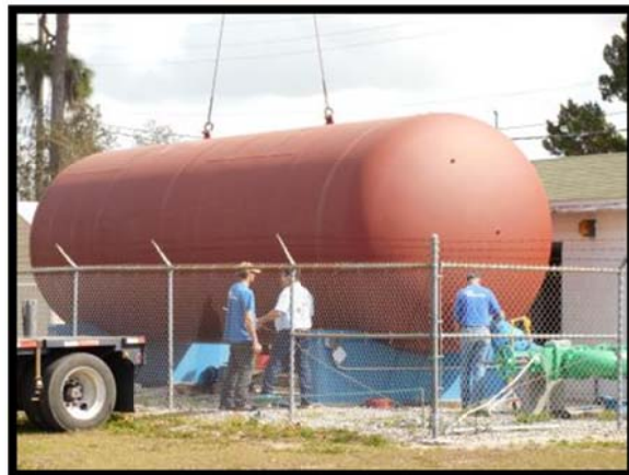
Installing new hydrotank.
