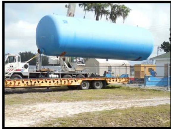
Installing new hydrotank.
