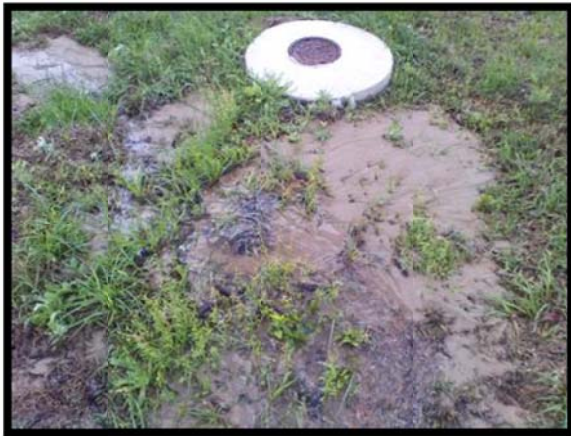
Leaking re-use main at Cardinal Hill WWTF.
