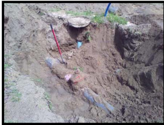
Leaking re-use main at Cardinal Hill WWTF.
