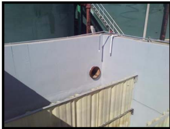
Re-sealing contact chamber at the Cardinal Hill WWTF.
