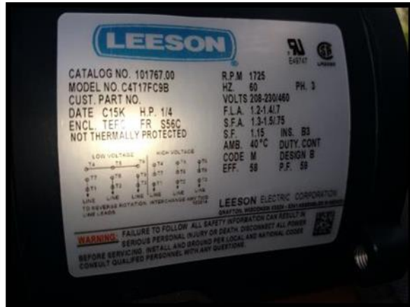
New motor for clarifier driver.
