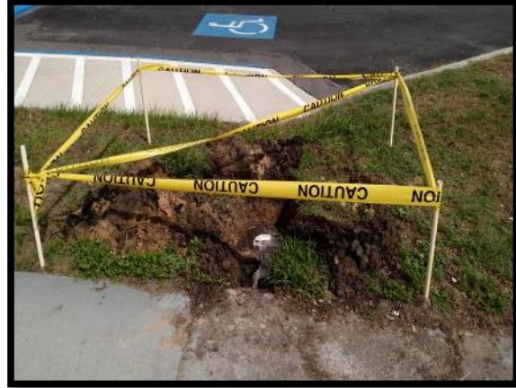
Two water line breaks.
