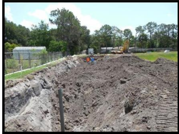
Sewer line replacement behind Duey Rd.
