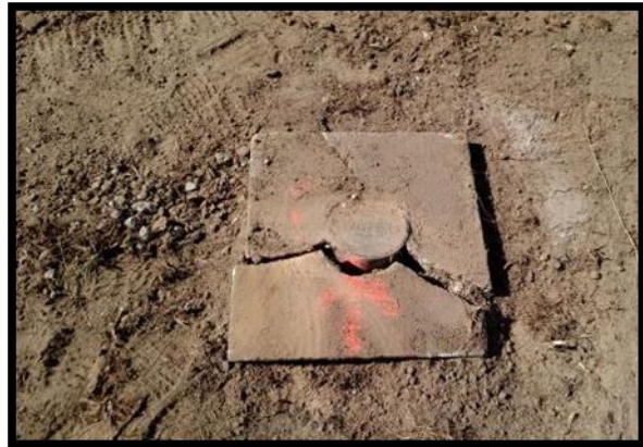
Broken valve box on Meandering Way.
